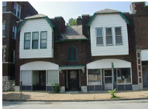
BEFORE: Existing transoms and projecting windows are covered with siding; Storefronts are inappropriate aluminum; Storm windows and door are inappropriate; Historic detail has been removed.
